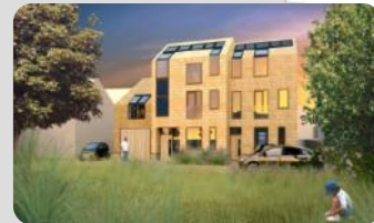
British Project Opening Q4 2010 Builder: VELUX
